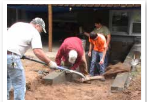
YouthBuild building a ramp for wheelchair access.
