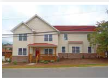
RCHA senior apartments in Davis, WV (top); Woodlands Development Group's (WDG) apartments in Mill Creek, WV, managed by RCHA (middle); WDG's LEED-certified Porter Street Apartments in Elkins, WV, managed by RCHA (bottom).
